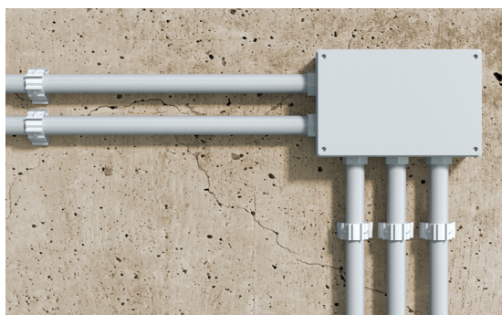
Fixing of cable clamps and junction boxes
